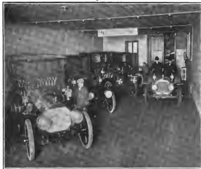
One upper floor of Stewart garage, cars in place
